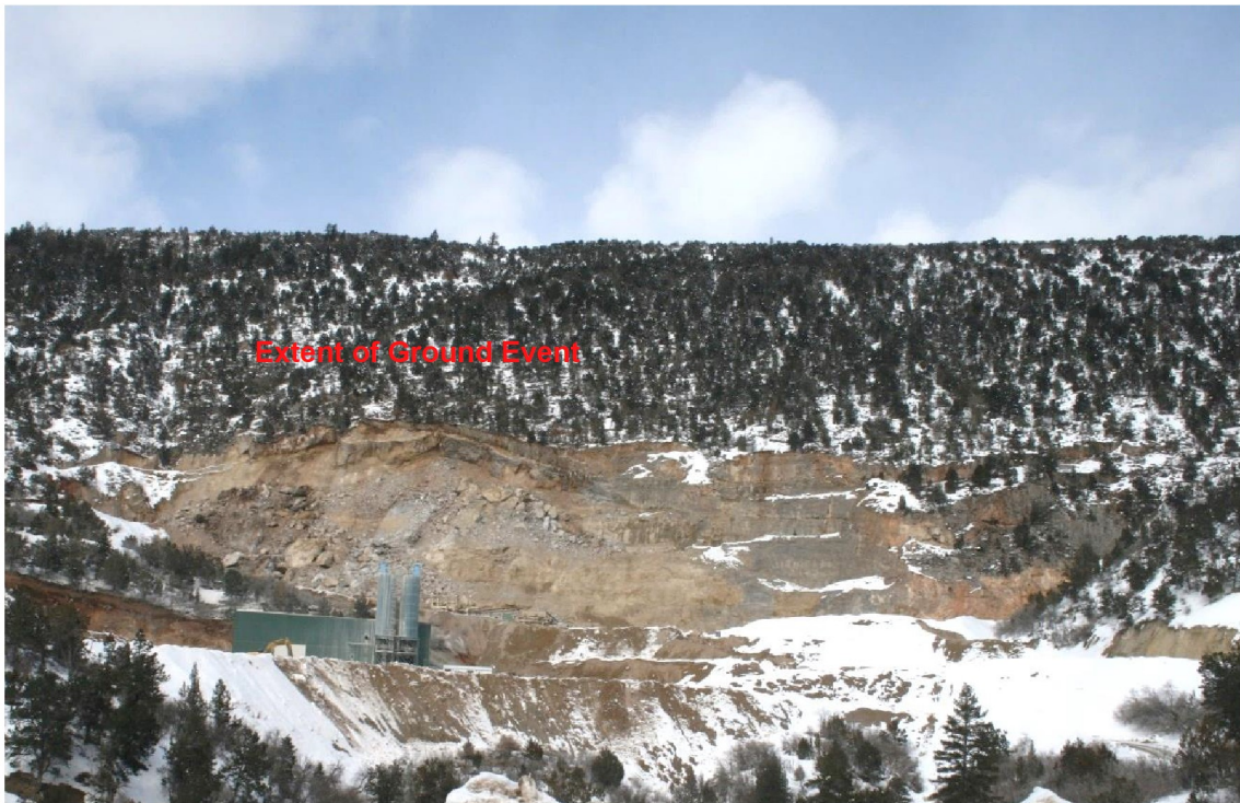
Photo 1: View of the Mid Continent Mine, west face on the left and East Face on the right. The January 2023 headwall ground event can be seen on the left, releasing on a consistent, NE-dipping joint plane. (1/26/23 Photo# 0613)
