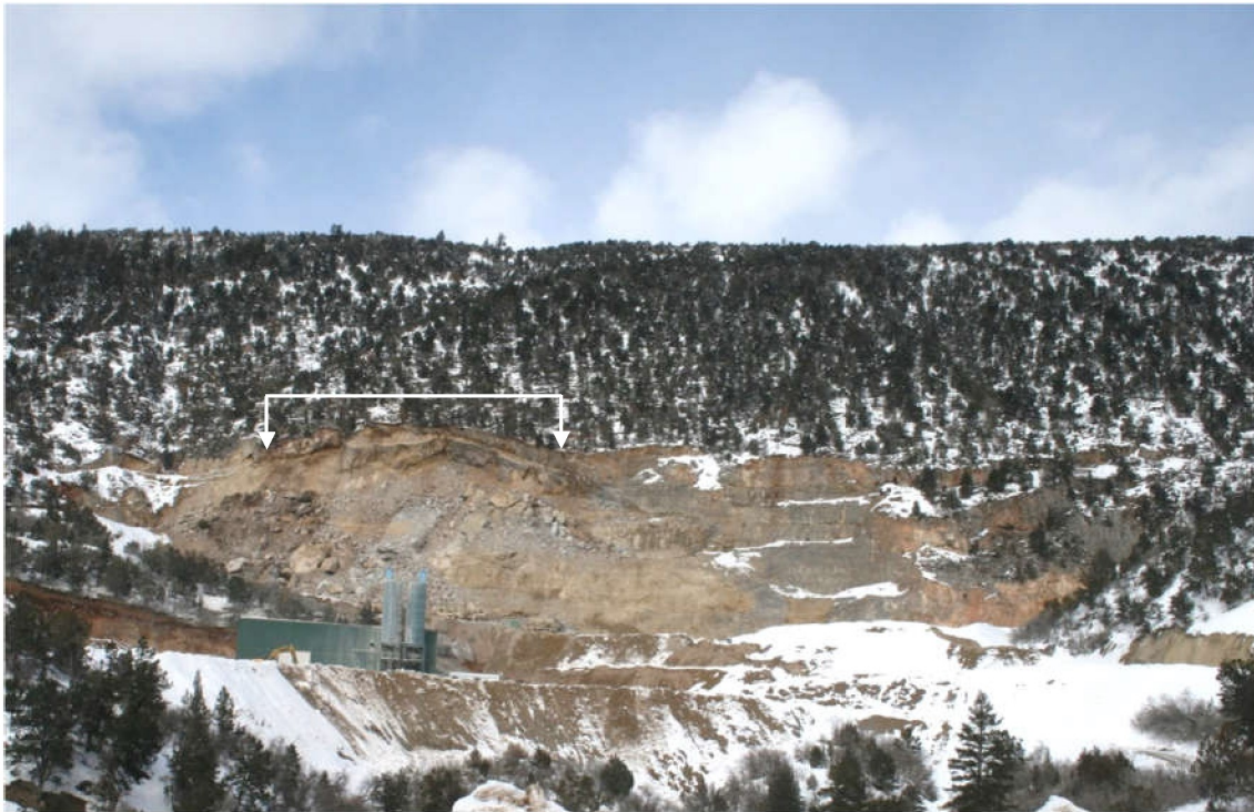
Photo 1: View of the Mid Continent Mine, west face on the left. The January 2023 headwall ground event (extent indicated by white arrows) released on a consistent, NE-dipping joint plane. (1/26/23 Photo# 0613)
