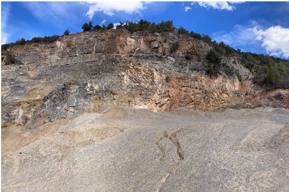
Photo 14: Looking up and north at the East Face. The bedding breaks defining the upper limestone beds are apparent. The East drainage on the right defines the eastern limit of operations. (4/14/23 Photo# 2002)
