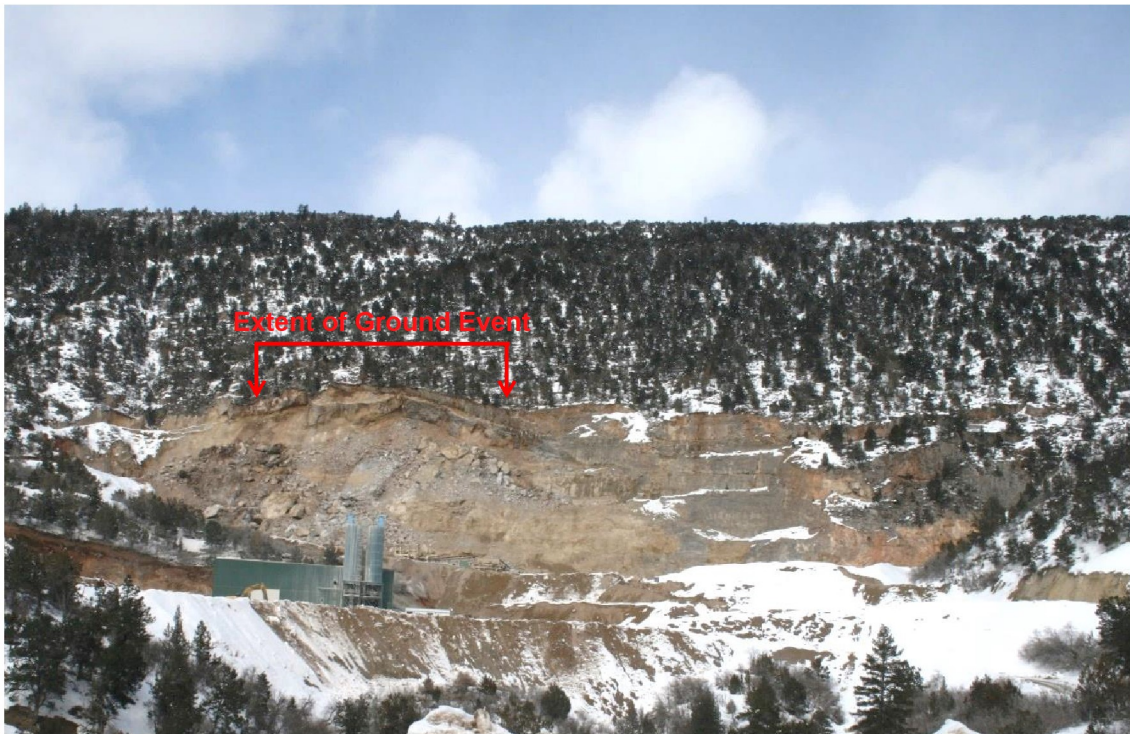
Photo 1: View of the Mid Continent Mine, west face on the left and East Face on the right. The January 2023 headwall ground event can be seen on the left, releasing on a consistent, NE-dipping joint plane. (1/26/23 Photo# 0613)
