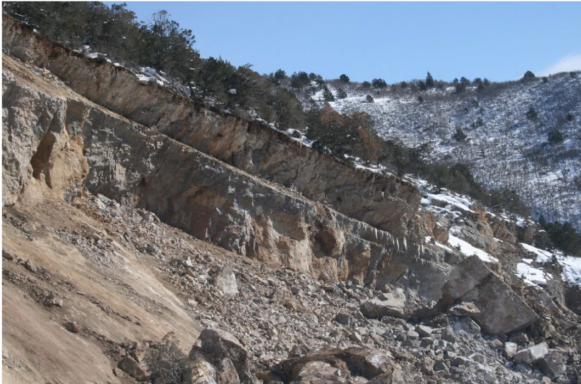
Photo 3: Side view, looking east, of the two upper units of the limestone with bedding acting as the slide plane. (1/26/23 Photo# 0598)
